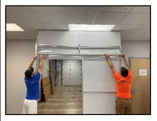
Next you will need to know your ceiling height in order to attach the correct extension panel to the adjustable top with the three provided splice bars. Slide 1 5/8" T-Nuts into the outer edge slot of the 1x2 door frame. Insert T-Nuts through the bottom of the adjustable top's predrilled hole (see below) then slide the top to the ceiling. Tighten knobs onto T-Nuts to hold
